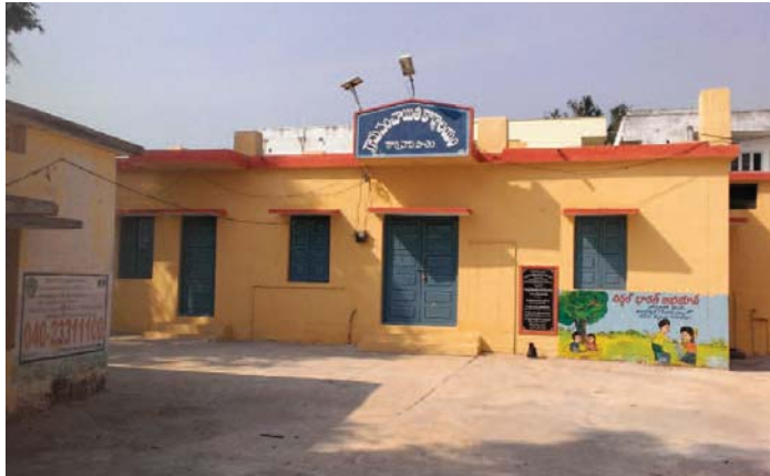
Gorlivanipalem Zilla Panchayat Office
