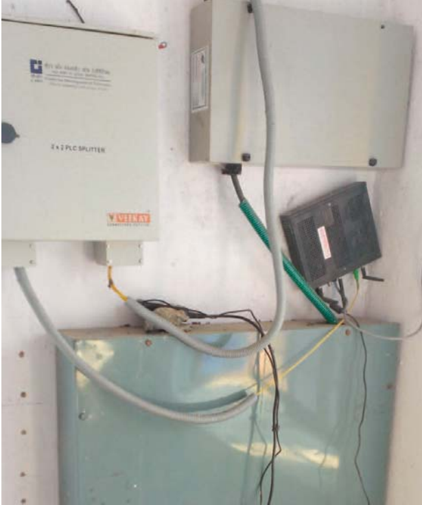
OFC (Optical Fibre Network) equipments in pilot locations
